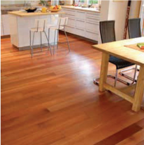
Solid Kempas Flooring finished with Osmo Polyx Oil.
