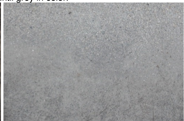
Clean Floor after Shot Blasting
