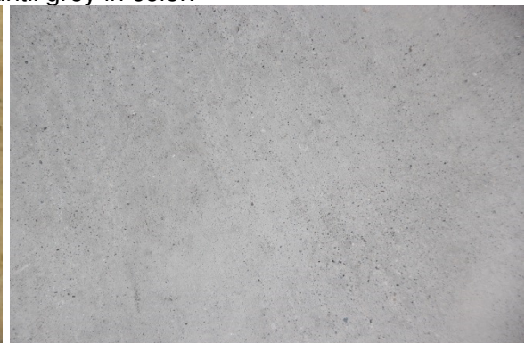
Clean Sub Floor
