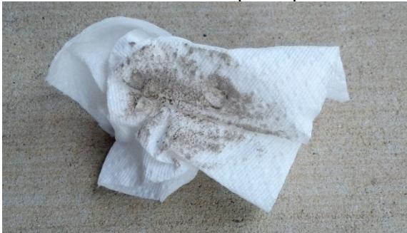
Dirt on Sub Floor
